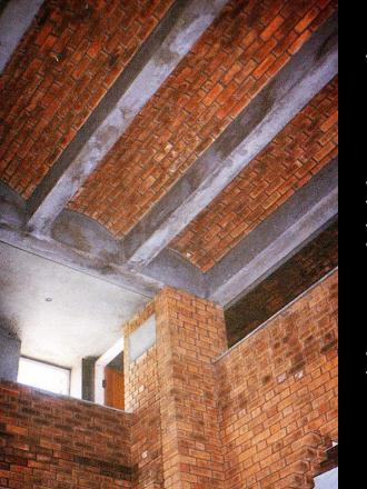
We have experimented with techniques like filler slabs, jack arch roofs, brick arches, brick vaults ,domes, rat-trap bond cavity walls, etc. which are not only cost effective & energy efficient but also make buildings sensitive to the climate.
