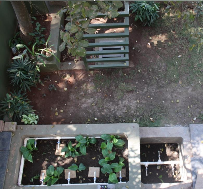
Waste water is recycled and is used for garden... Earth tunnel is provided to cool air inside the building...
