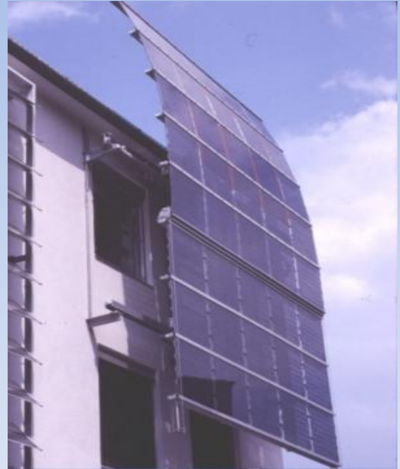
Movable solar shading device, made of transparent modules (Photo: Denis Lenardic)
