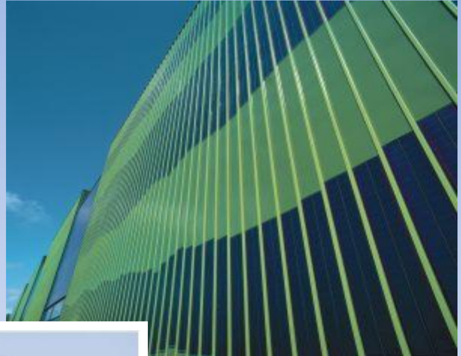
Large transparent module - glass/glass laminate (courtesy Ertex Solar GmbH ).
