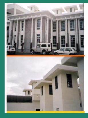
Passive Downdraft Evaporative Cooling (PDEC) System
